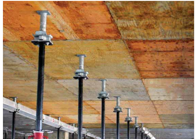
Framing Members Removed
